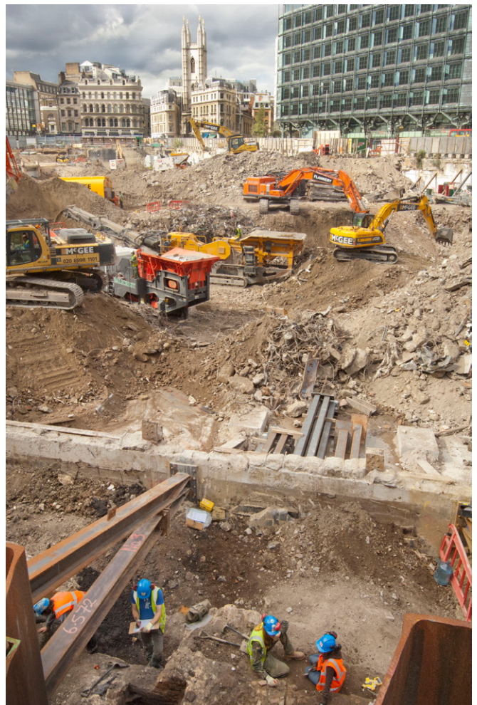
The excavation at the site of Bloomberg's new building. © MOLA
