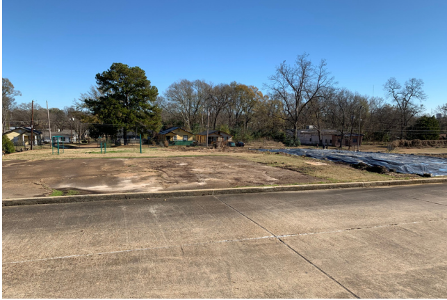
Galloway Elementary Pre-Installation Photo
