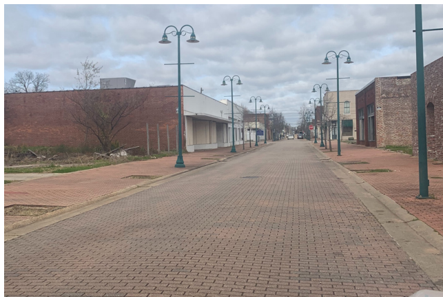
Farish Street Pre-Installation Photo
