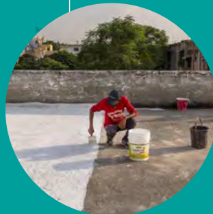
Ghaziabad, India Converting cow dung into white rooftop paint that cools homes, lowers emissions, and creates jobs for women who produce the paint.
