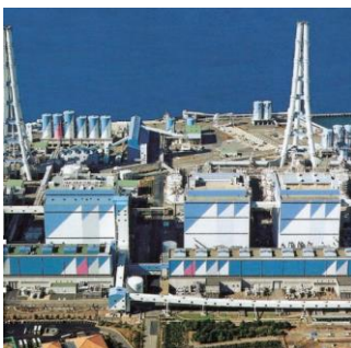
Figure 5: Jera's Hekinan coal-fired power plant
